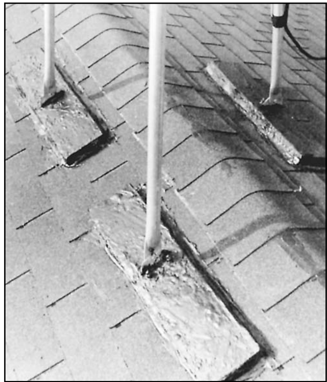
Fig 45— Three lengths of 2 x 6 wood mounted on the outside of the roof and reinforced under the roof by three identical lengths provide a durable means for anchoring the tripod. A thick coat of roofing tar guards against weathering and leaks.
