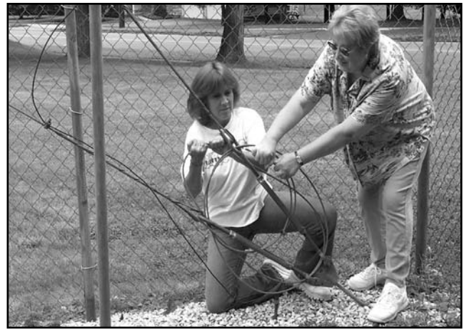
Fig 24 —A length of guy cable is used to assure that the turnbuckles remain in place after they are tightened. This procedure is an absolute requirement in guyed tower systems. (Photo by N4QX)
