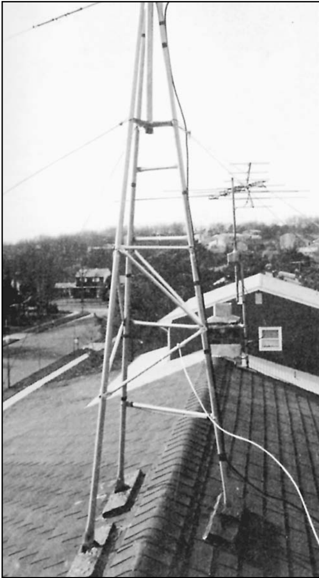
Fig 43— This tripod tower supports a rotary beam antenna. In addition to saving yard space, a roof-mounted tower can be more economical than a ground-mounted tower. A ground lead fastened to the lower part of the frame is for lightning protection. The rotator control cable and the coaxial line are dressed along two of the legs. (Photo courtesy of Jane Wolfert.)
