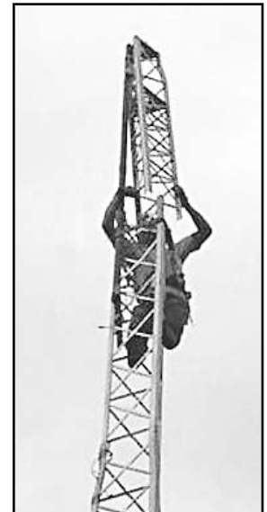
Fig 22—Climber is guiding the new section onto the top of the existing one. The gin pole attached to the left leg is bearing the weight, as the climber gives verbal instructions to the ground crew pulling on the gin-pole rope. (Photo courtesy Mike Hammer, N2VR.)
